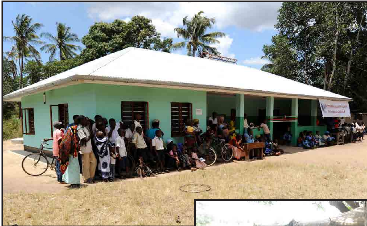
Villagers gather around the newly renovated Masaika Health Clinic in the Pangani District of Tanzania during a dedication ceremony, October 2009. The clinic provides outpatient service to a community of more than 1,800 people and (left)
